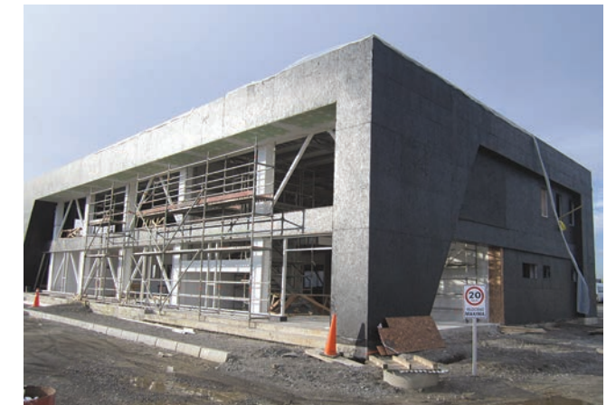
The project is now well underway
