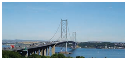
The Forth Road Bridge in Scotland
